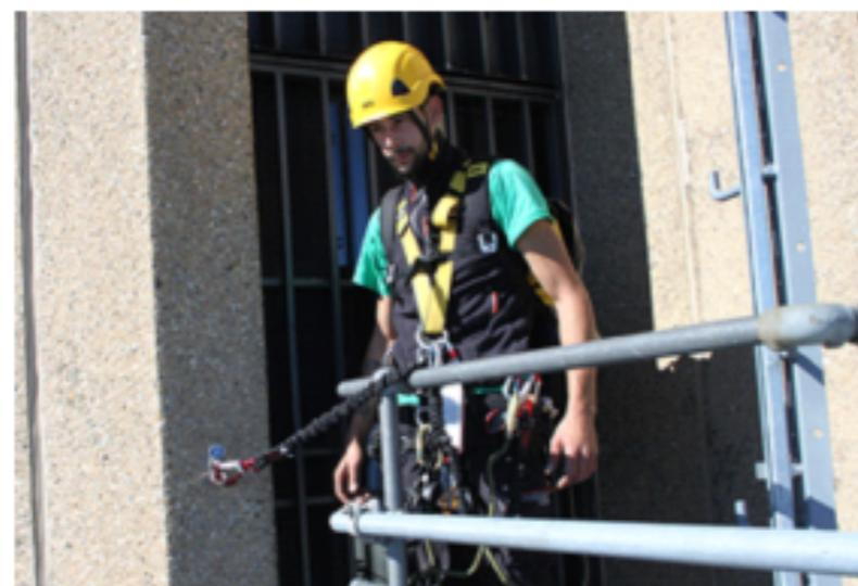
The operator can access the roof from the internal part of the building and must walk through an area with parapet. The operator must anchor himself to the eye bolt Infinity I using an Y-lanyard with energy absorber (EN 355) and access the roof.
